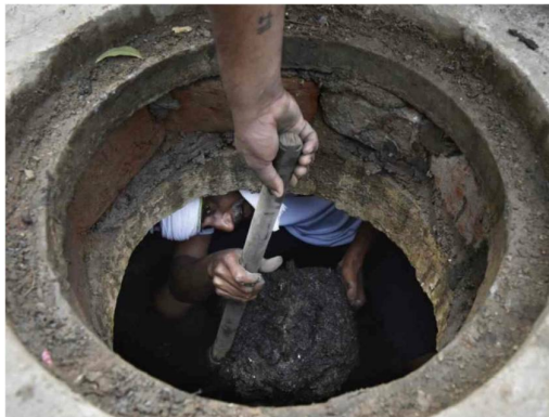
Figure 3.1 Workers In Drainage
